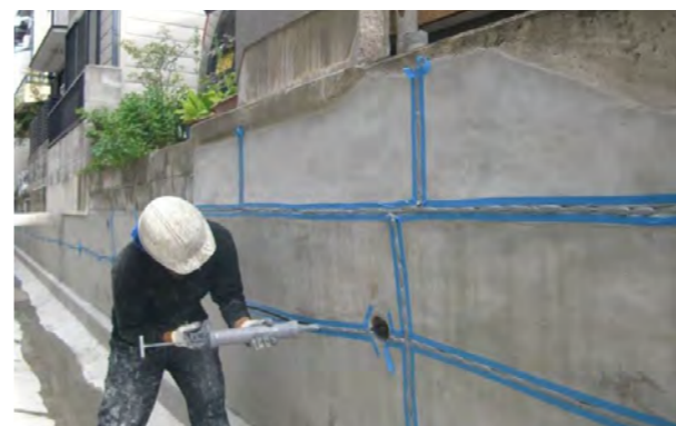
③ ひび割れ補修工
