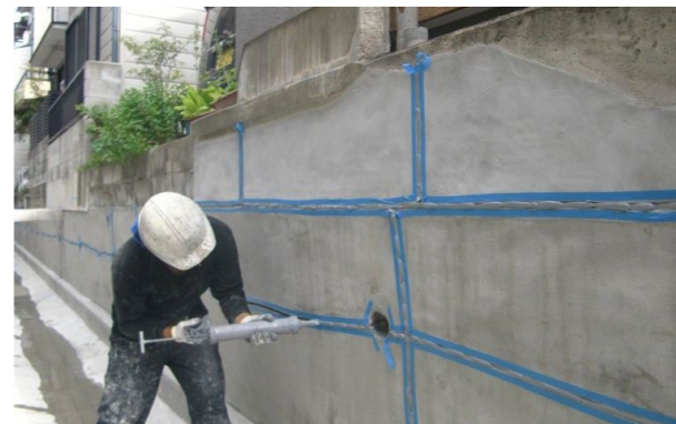
③ ひび割れ補修工
